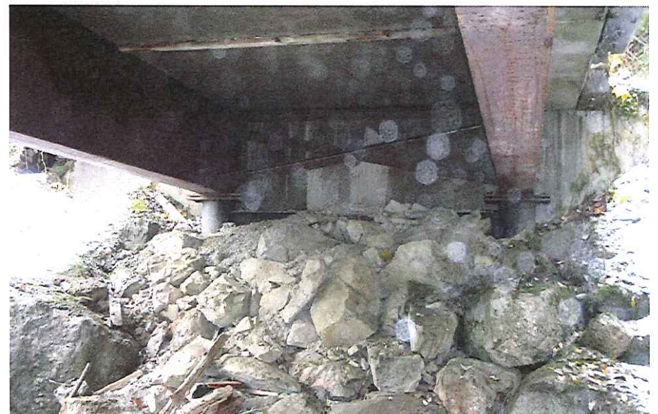
CK-2024 Abutment Right Bank
