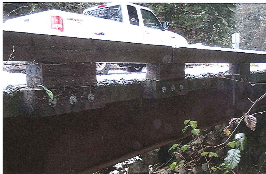
CK-2024 Crossing Upstream
