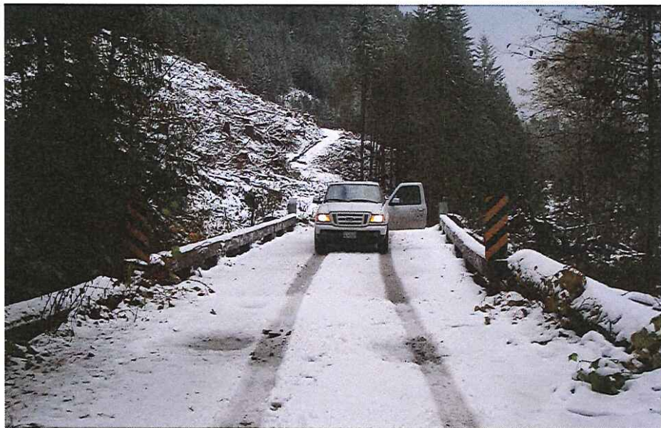
CK-2024 Approach Right Bank
