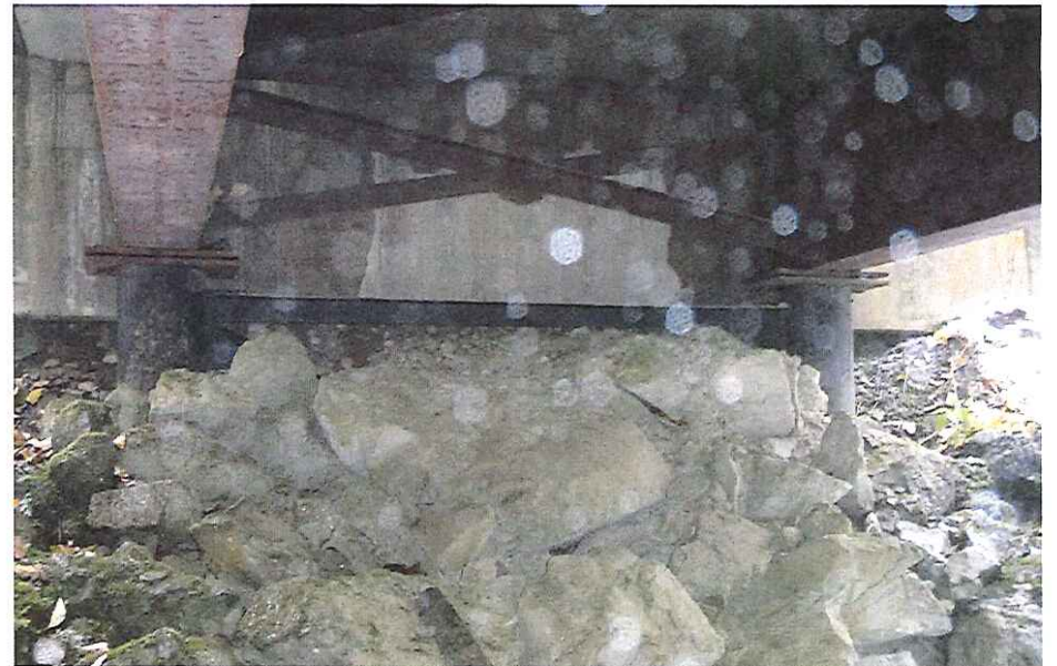
CK-2024 Abutment Left Bank
